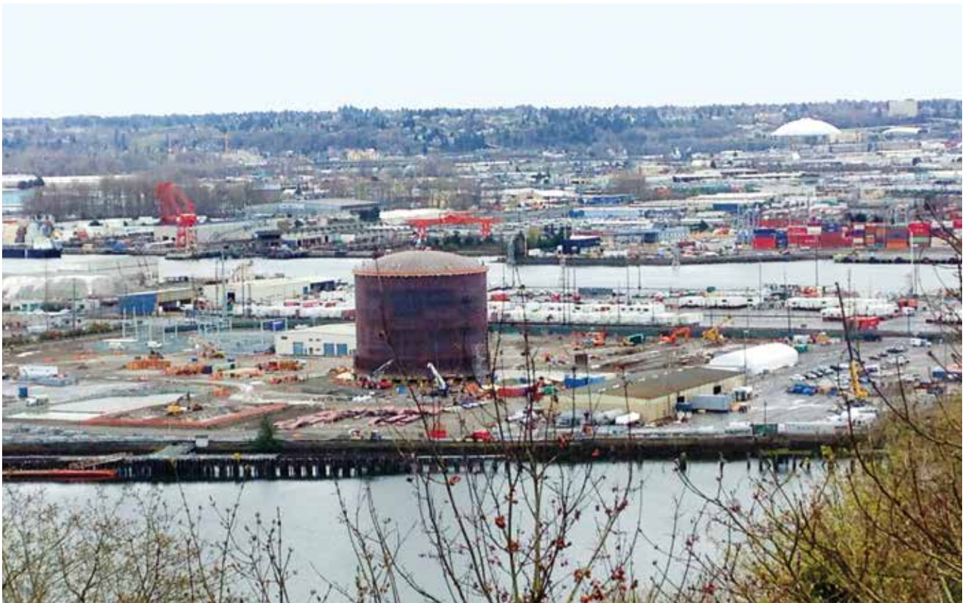
The Tacoma LNG facility under construction
